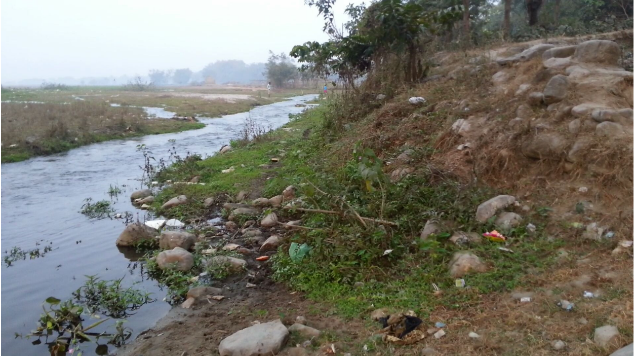
Photo-6: Partly Eroded abutment spill due to attack of active channel
