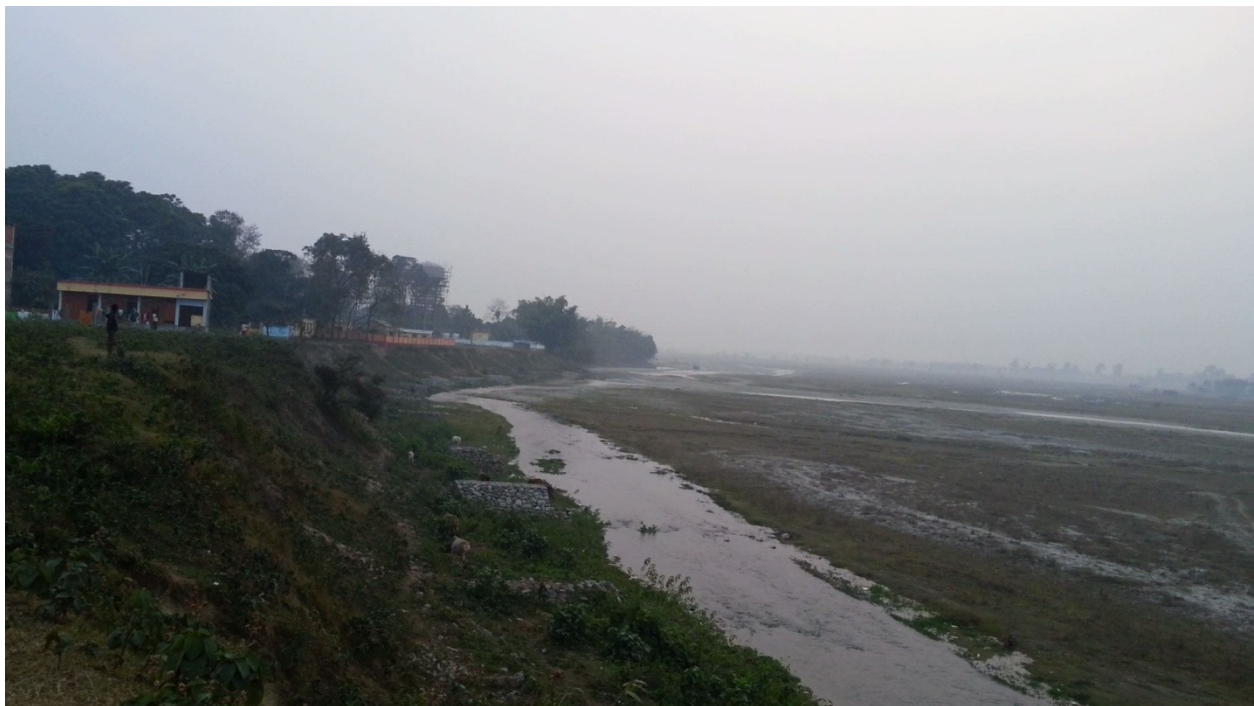
Photo-4: Showing downstream bend and deep erosion
