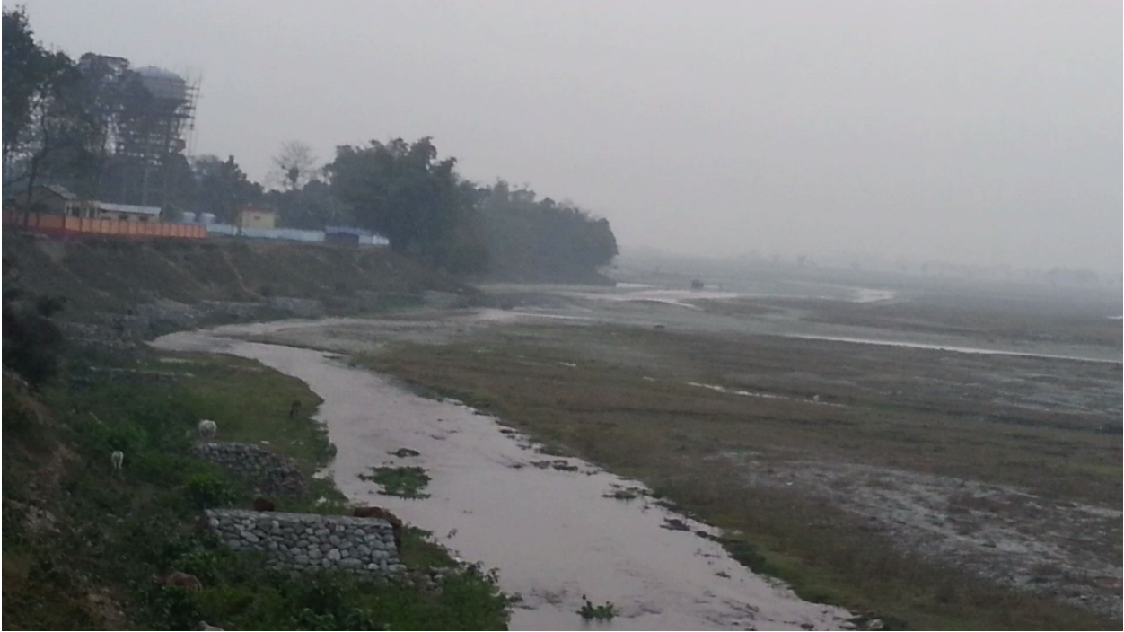
Photo-6: Partly Eroded abutment spill due to attack of active channel
